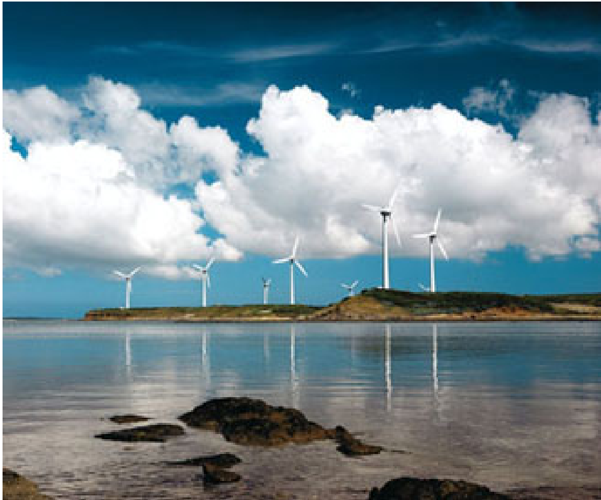
A wind farm built by Taipower in Baisha Township of outlying Penghu County (Photo courtesy of Taiwan Power Co.)
