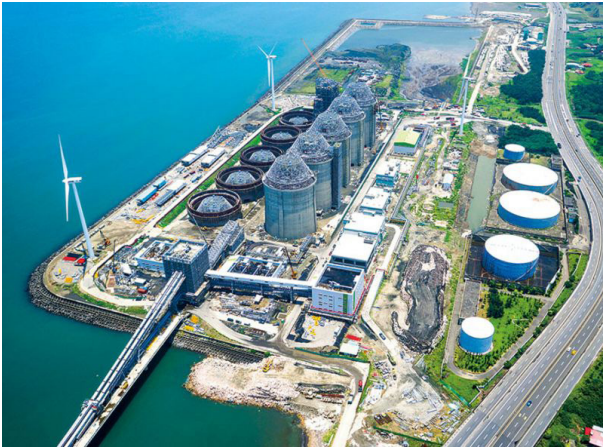
New Taipei City's Linkou Power Plant began operating Taiwan's first ultra-supercritical coal-fired generator in October 2016. (Photo courtesy of Taiwan Power Co.)
