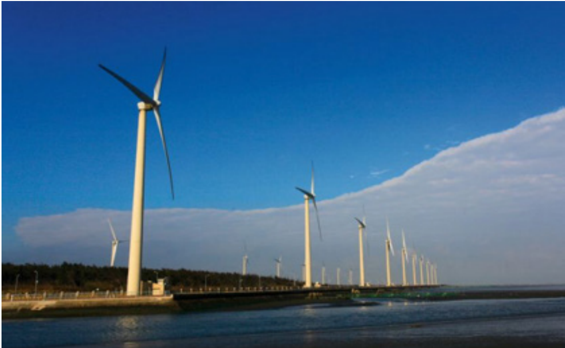
State-owned utility Taiwan Power Co. operates wind farms in the Gaomei Wetlands of central Taiwan's Taichung City. (Photo by Jimmy Lin)
