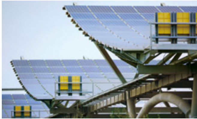
Magong Airport in offshore Penghu County is equipped with solar power facilities. (Photo by Chin Hung-hao)
